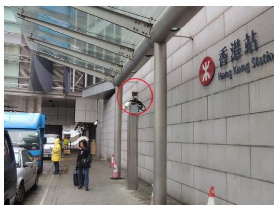
A camera installed at the passenger drop-off areas in Hong Kong Station.
